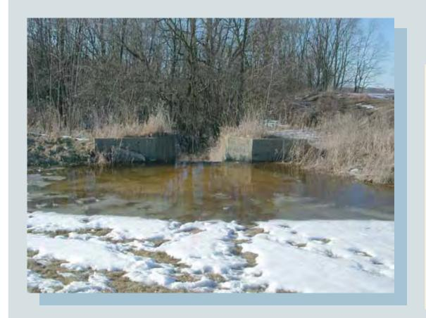
The concrete chute spillway consists of an inlet with wing walls, a vertical curve section, steep-sloped rectangular open channel, velocity check (the triangular concrete piece), stilling basin, and outlet. Flowing water is concentrated and accelerates down the channel then is slowed at the bottom by turbulence created by the velocity check and basin, thereby minimizing soil erosion.
