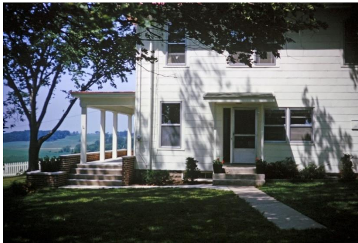
Lower level is remodeled, and new entrance added.
