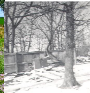
Remnant of the old carriage shed in disrepair. (1962)
