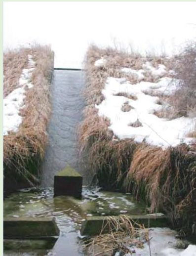
Spillway still works in 2020.
