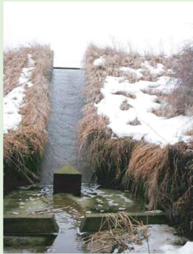
Spillway still works in 2020.
